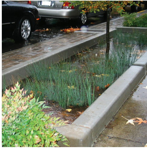
Bioswales provided at the street edge reveal and celebrate stormwater filtration.
