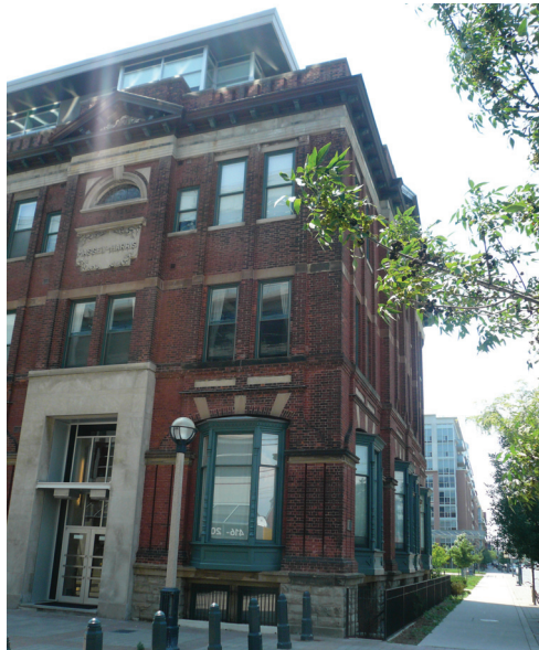
An example of adaptive reuse where an existing building was redeveloped, while maintaining the original building structure, and adding new construction on the roof.
